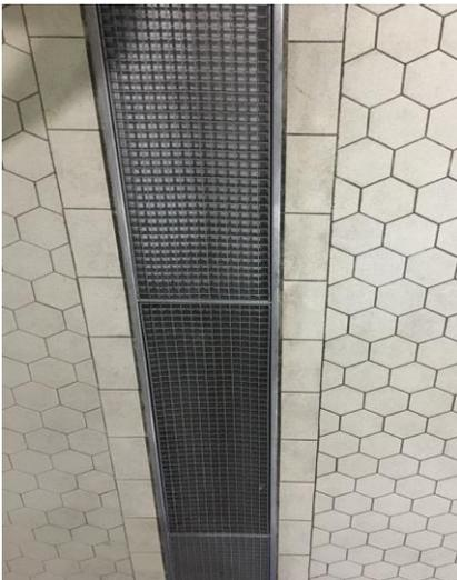
**Figure 4 : Anti-slip tiles flooring (R10-R11)**
